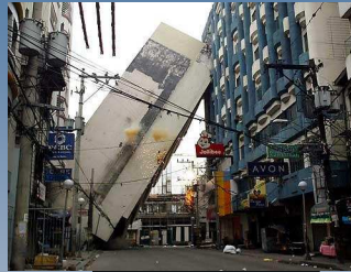
Poor Quality Infrastructure
